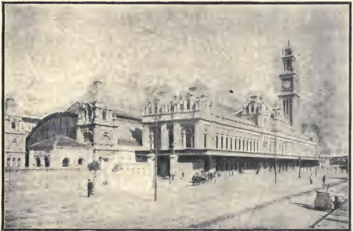
FIG. 189—Railroad Station, Sao Paulo, Brazil
